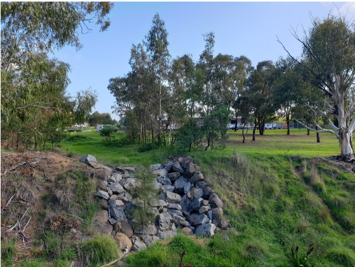
Figure 60: BRC PP3 - Across Creek to North - 23 March 2020
