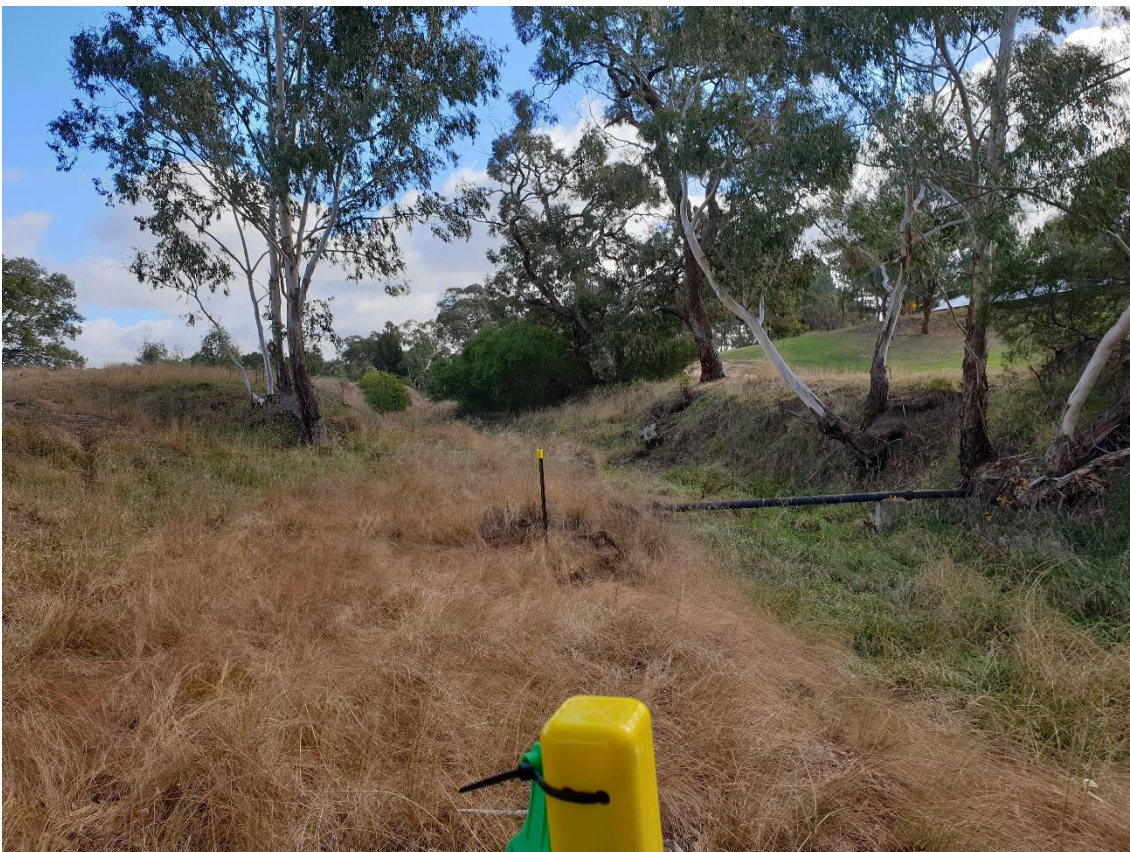
Figure 6: Photo Point 1 - Upstream - 30 May 2019
