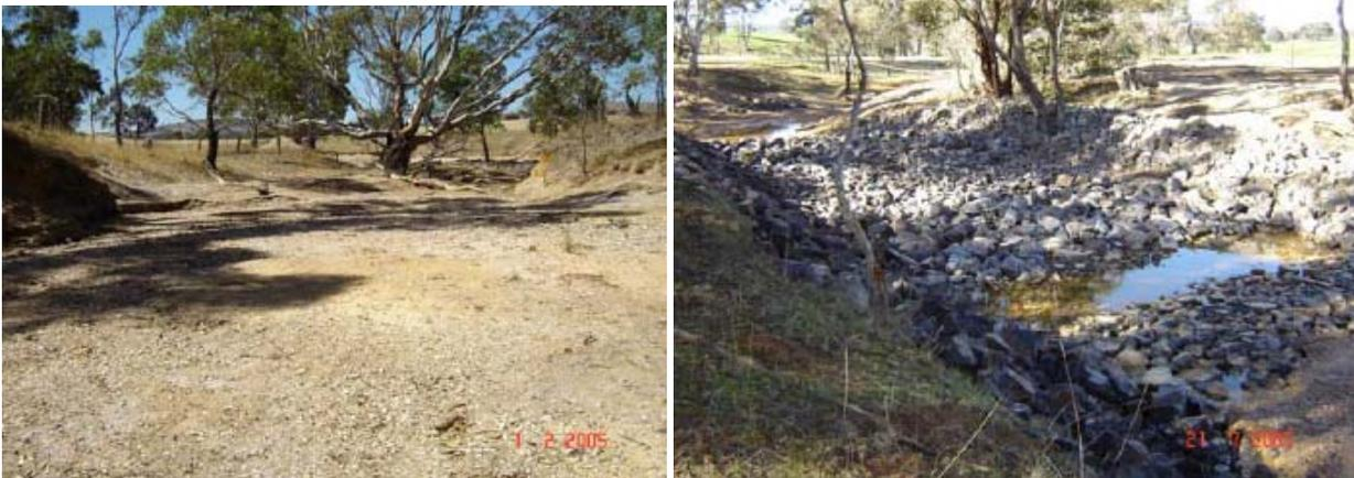
**Figure 4. Before and after – 'Elevated Crest' rock chute.**
