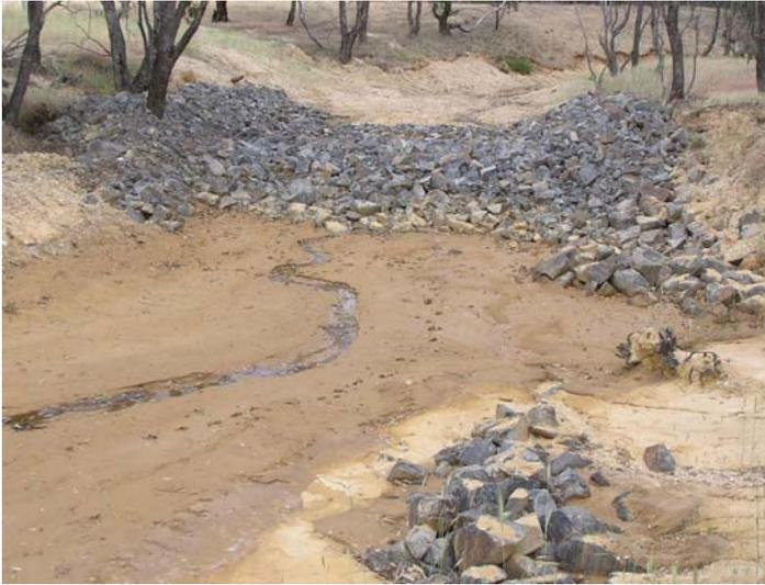
**Figure 3. Evidence of sediment build up and storage on upstream side of existing rock chute.**
