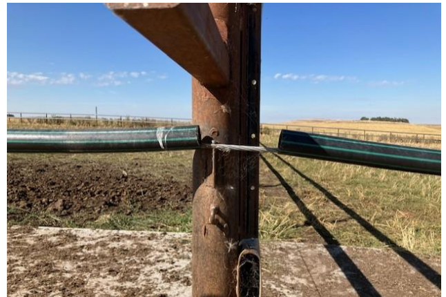
Figure 6. Poly pipe covering on cable (close-up).
