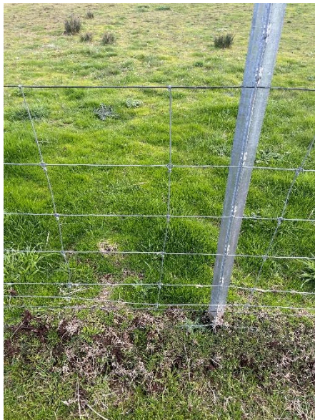
Figure 3. Clipex fence post and 7/82/30 ringlock
