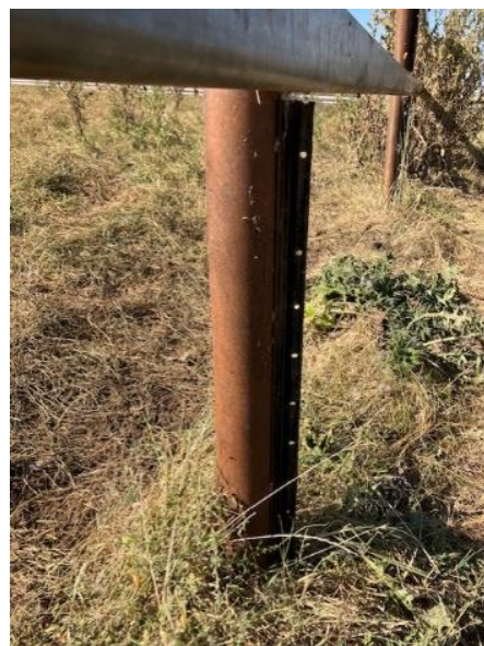
Figure 7. Star post welded so additional wires can be run if needed.
