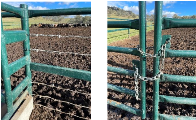
Figures 7 & 8. Rails, cable and gate latches used in construction
