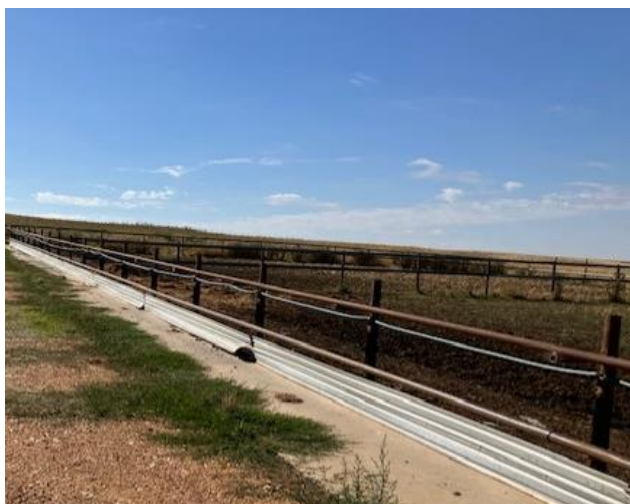
Figure 5. Poly pipe covering on cable.
