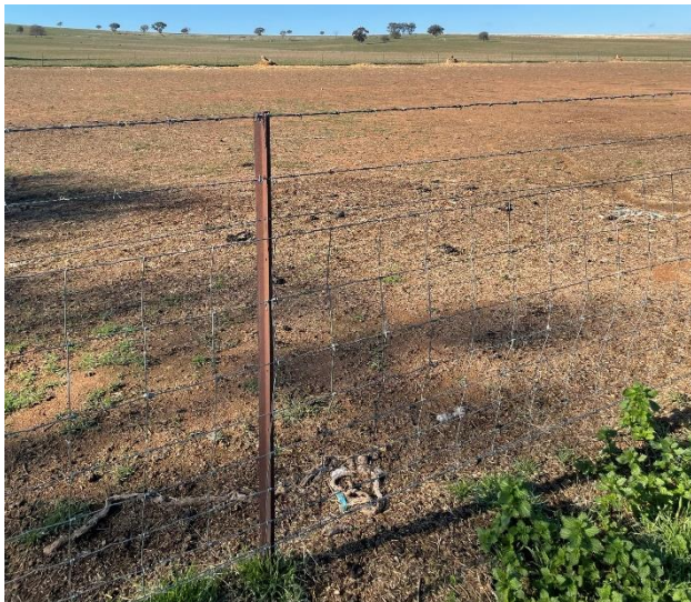
Figure 3. Steel posts, ringlock and barbed wires used
