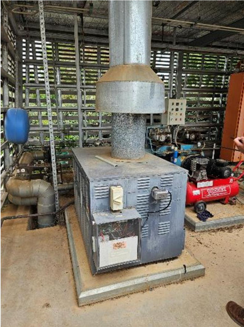
B295 Boiler – 225kW (70°C)
