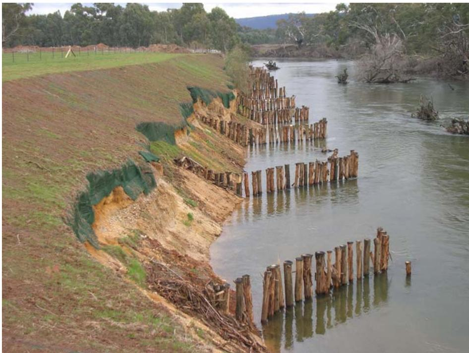
**Figure 2. A timber pile field site constructed on the Murray River in 2006.**
