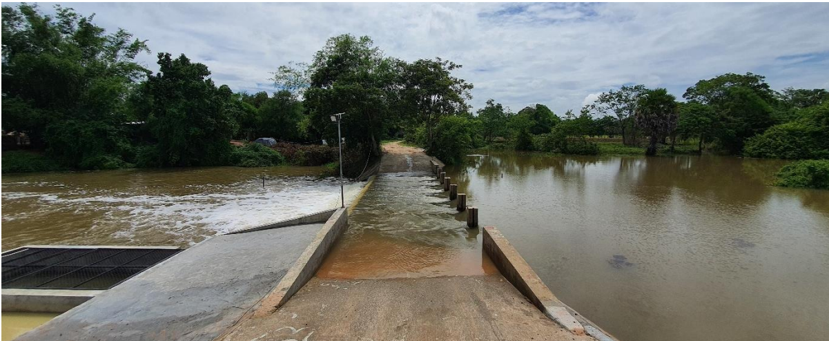
Photo 3. Sleng fishway site without handrail across the spillway
