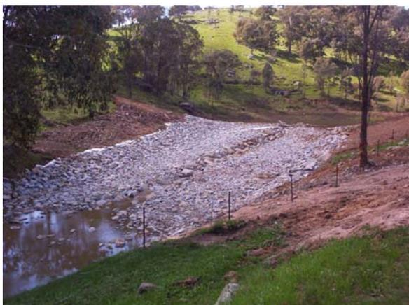
**Figure 5. Main chute with completed fishway.**
