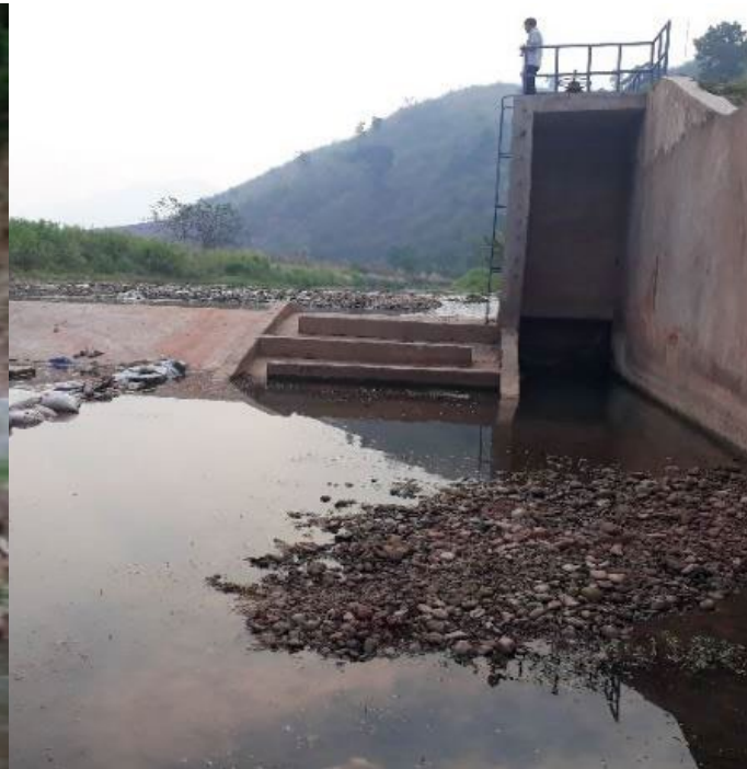
Improperly Designed Fish Ladder
