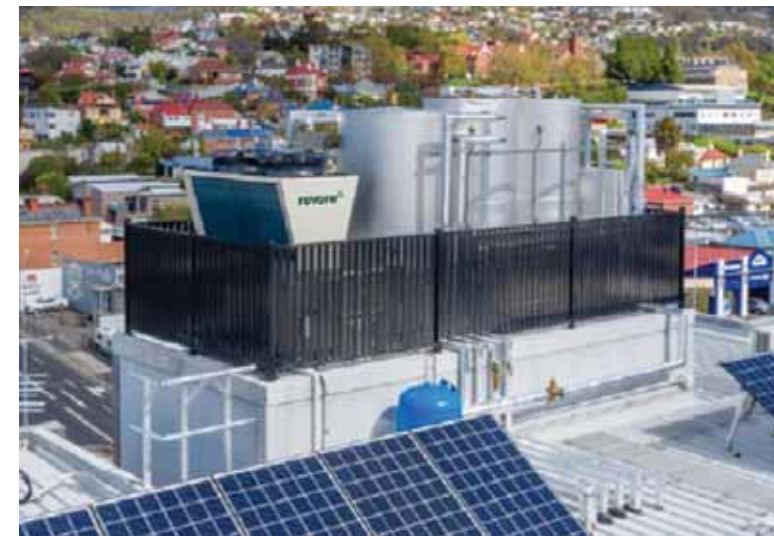
1 x Revere CO2 76kW Heat Pump w/ 2 x 500L DHW tanks (1,000L) & 1 x 800L HHW buffer tank ($110k/skid)
