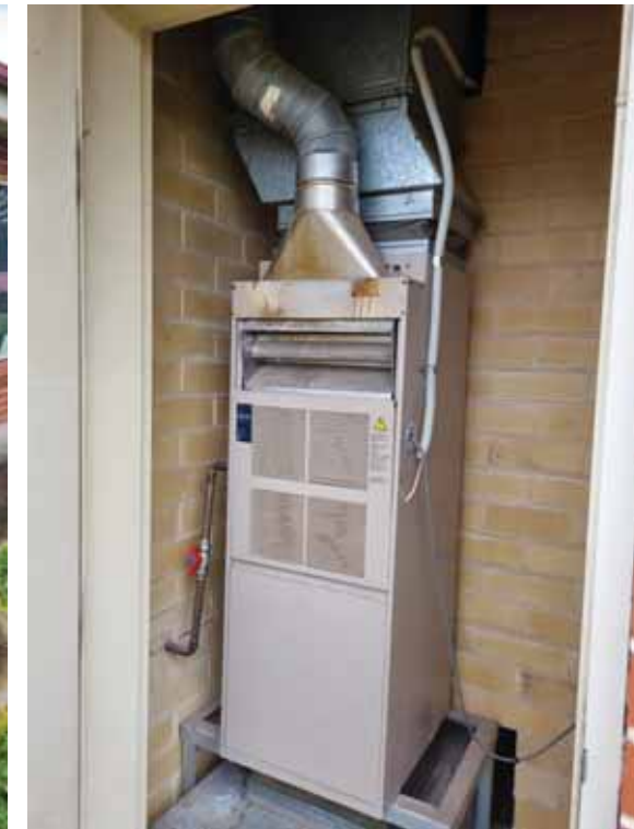
Diggings – ducted gas heating system
