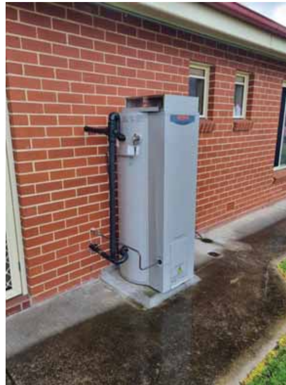
Diggings - Gas hot water system
