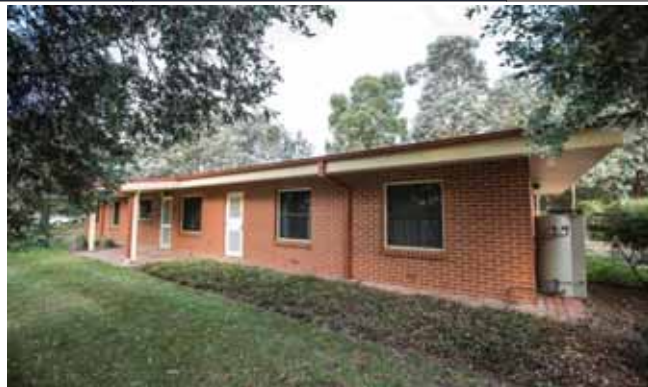
Windradyne – Gas storage system
