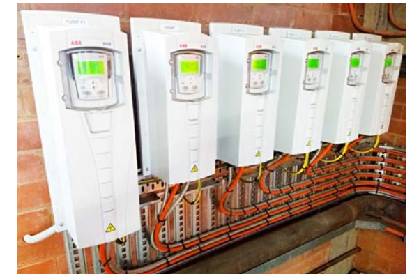
Installation of variable speed drives
