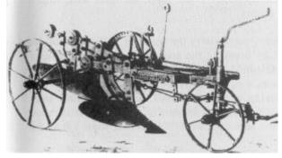
Figure 1.3 Early stump-jump plough invented by R.B. Smith of South Australia in 1876; this implement was especially useful in Mallee country
