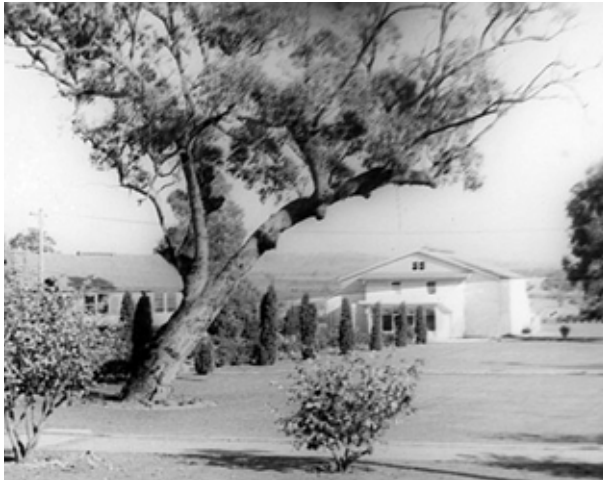
Figure 14 Auditorium: long view with garden, 1970s
