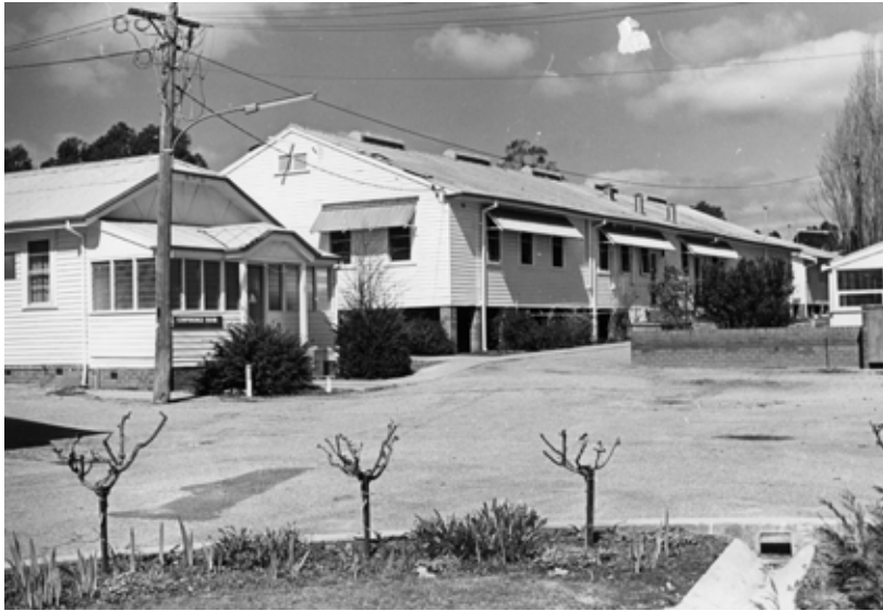
Figure 7 Conference room and Creative Arts building, 1970s
