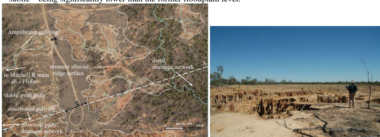
Figure 1. (Left) Example of amphitheatre gully form on the mid Mitchell River. Figure 2. (Right) On ground photo of the same general area. Note how the gullies are progressing towards the highest ground (as represented by the remnant alluvial ridge surface – depicted by the loop road) from both sides, and the very small “upslope” contributing catchment area adjacent to each gully (indicated with the arrows 1 and 2).
