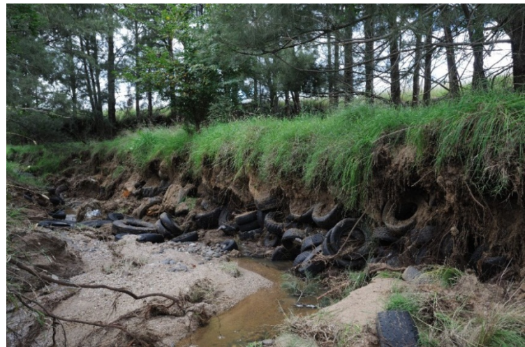
Plate 12. Broken tyre wall overplanted with River Sheoaks
