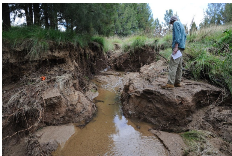
Plate 10. Active erosion in Hawthornden Creek following heavy rain in February – March, 2012.
